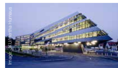
The Institute of Structural Lightweight Design is located in Science Park 1.
